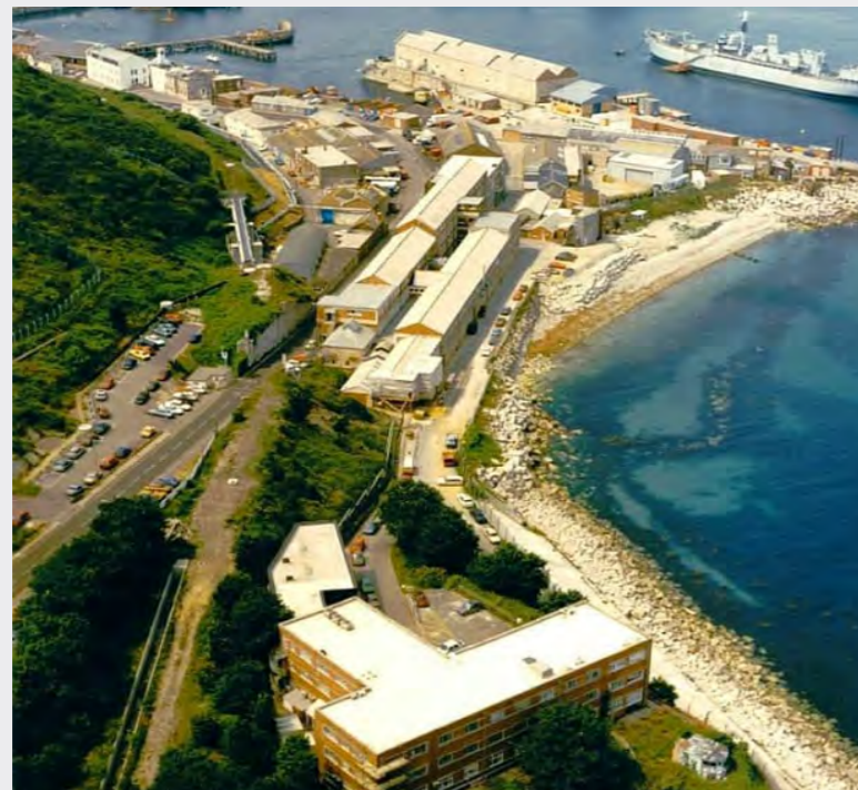
Aerial view from the south showing the HM Underwater Detection Establishment "North" and "South" buildings that were demolished in 2005.
