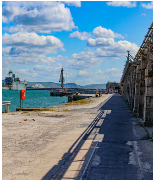
50T crane birth and arches of the Inner Breakwater (private view)
